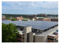
By collaborating to install **solar panel canopies** on the Regents Drive, Terrapin Trail, and Mowatt Lane parking garages, the Department of Engineering & Energy in Facilities Management and the Department of Transportation Services helped increase campus solar energy production capacity by around 200% to reach almost **3 megawatts** The project supports the President's Purchased Power Initiative to ensure 100% of purchased power comes from renewable sources by 2020.
