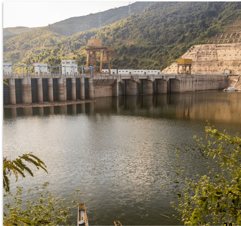
Nam Long Hydropower Project, Laos
